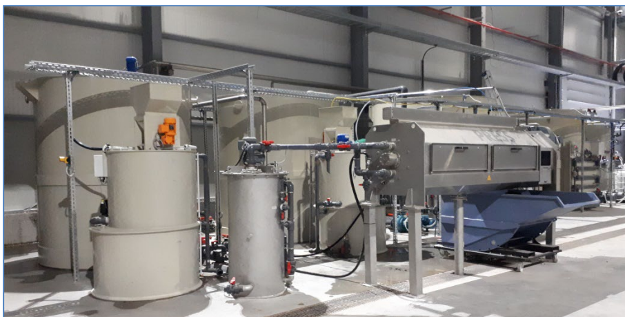
Figure 16: Extended Water Treatment
